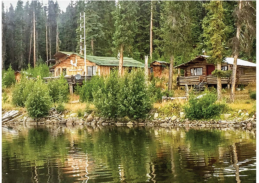
Built in 1986, when we first approached Eliguk it looked like an abandoned town.
